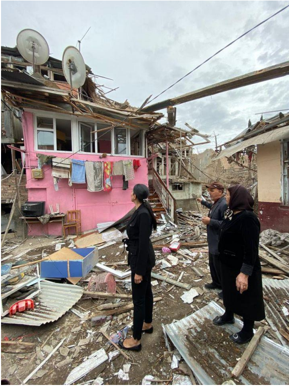
Destroyed private house – Photo 4.
