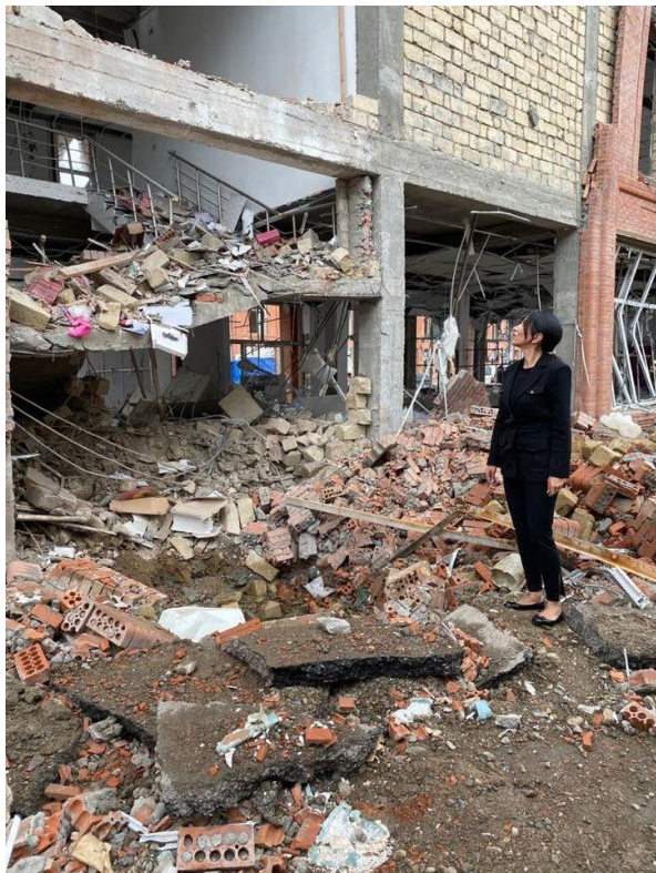
Destroyed shopping center - Photo 7.
